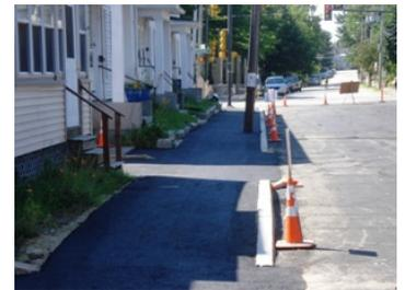
Continental Paving has graded and base paved a portion of sidewalks on North Spring Street. They will finish grade and base pave the rest of the sidewalks next week. They will also start raising the catch basins and manholes in preparation for the final overlay.
