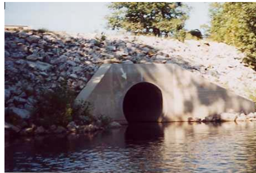
Outfall on the Merrimack River
